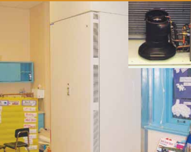
An optional sound-deadening compressor jacket and sound-attenuating door helped LAUSD achieve noise levels below 45 dBa.
